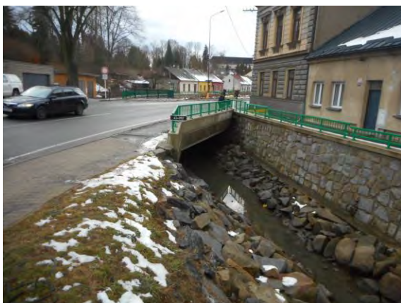
Mostek km 93,097 - pohled po toku na most
