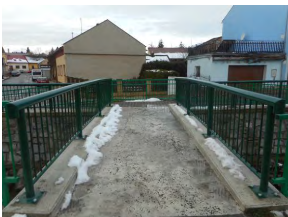
Mostek km 93,280 - detail
